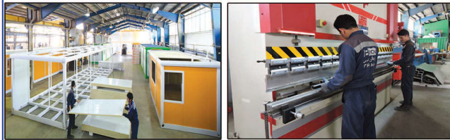
EPS parts production line. (sheets and parts)
